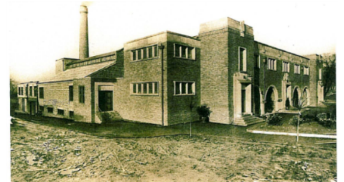
THE HEATH TOWN PUBLIC BATHS, WASH-HOUSE AND LIBRARY BUILDINGS
